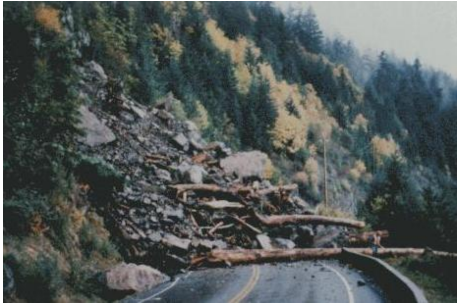
Figure 1 In 1991, a rock slide near Loggers Creek closed the Sea-to-Sky Highway for 12 days and cost $7 million for repairs and preventative structures (photo courtesy of the Ministry of Transportation and Highways).
