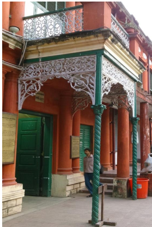
Figure4 Use of wrought iron posts and facia in porch of a Heritage building at Dalhousie square
