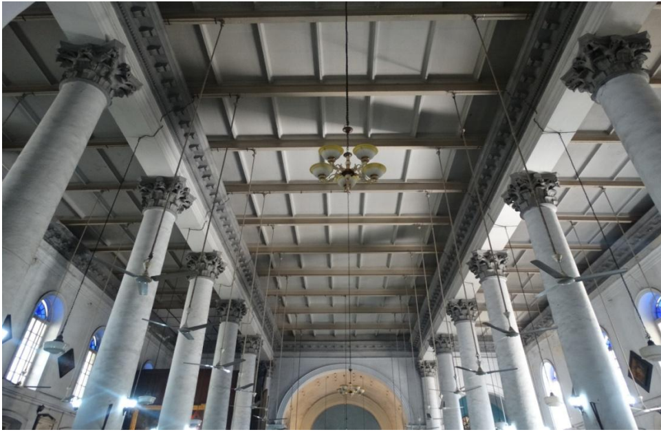
Figure3 Use of structural steel in Church at Dalhousie Square
