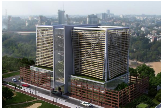
Figure5 Volvo Eicher Building
