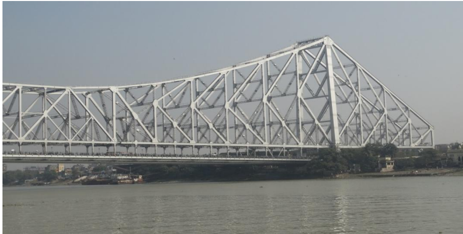
Figure1 Howrah Bridge "Ravindra Setu"
