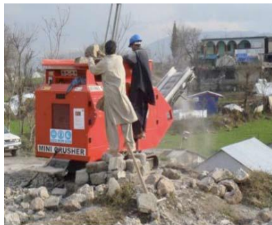
Fig-5 Crushing building wastes
