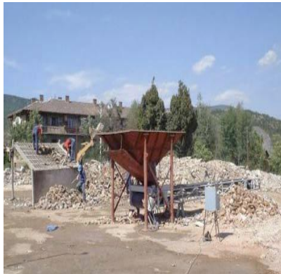
Fig-3 Sorts finer material from over size concrete
