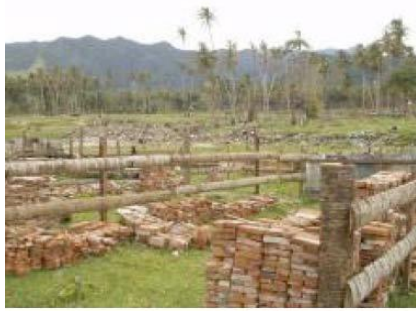
Fig-1 Stacked cleaned bricks for re-use
