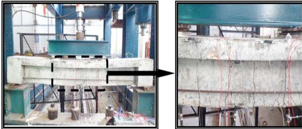
Fig. (8) Crack pattern for specimen MD0 S 2.8-26%
