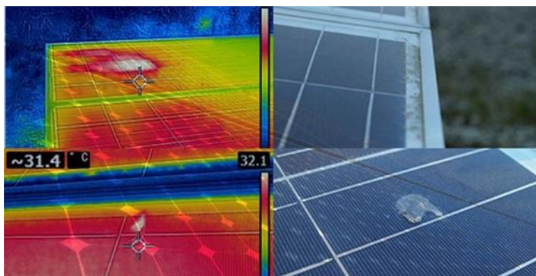
Fig. 1 Solar panels that emit effects from Hot Spots
