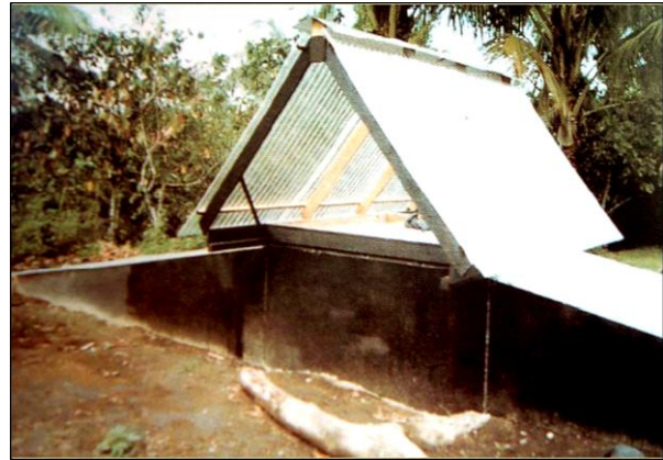
Diagram 7: Showing shows solar dryer with central rock solar collectors and polycarbonate sheet roof
