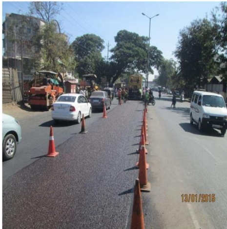
Microsurfacing Laying
