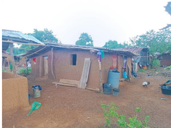
Plate 1: Pictorial View of mud used in the construction of walls. Source: Author's fieldwork; May, 2024.
