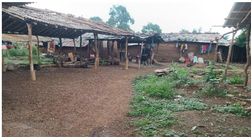
Plate 4: Pictorial View of wood used in the construction of posts for the kitchen and the outdoor sheds. Source: Author's fieldwork; May 2024.
