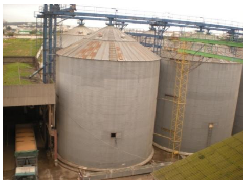
Fig. 1 Metal storage infrastructure of grain silo
